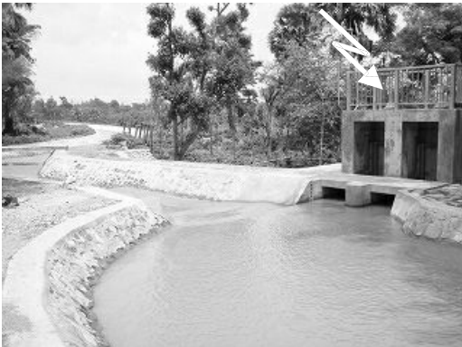
Sediment settling basin (2)
